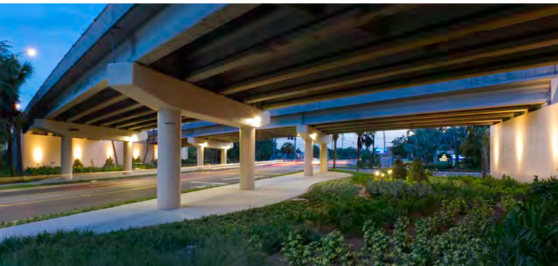
Selmon Expressway overpass at Swann Avenue
