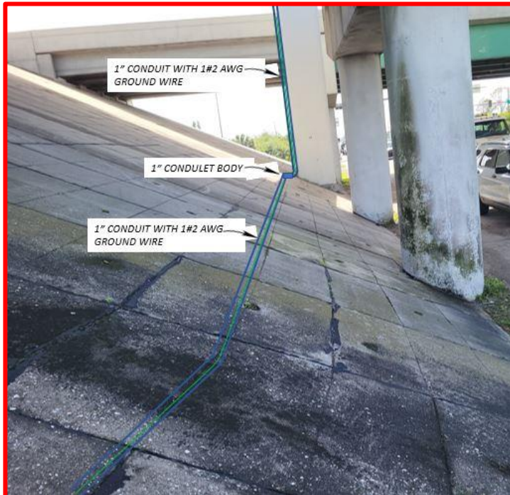
Figure 11B. Horizontal Conduit on Slope Pavement
